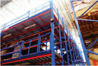
Rack Support Mezzanine floor
